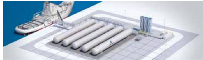
■ Fig. 4 - Small-size LNG terminal based on insulated bullet tanks. Ideal for: smaller-size terminals where a storage capacity up to 15,000 m 3 is required or where there is not sufficient availability of local labour and construction equipment. Advantage: a solution that needs minimal site work, as most of the work is shifted to factories.
