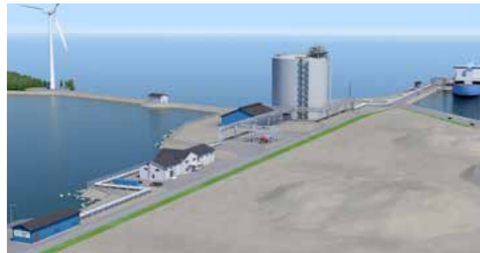
■ Fig. 3 - Medium-size LNG terminal based on a flat-bottom concrete tank. Ideal for: terminals where a storage capacity over 15,000 m 3 is required and where local labour and construction equipment are available. Advantage: a well-insulated tank and terminal that can withstand any type of weather.
