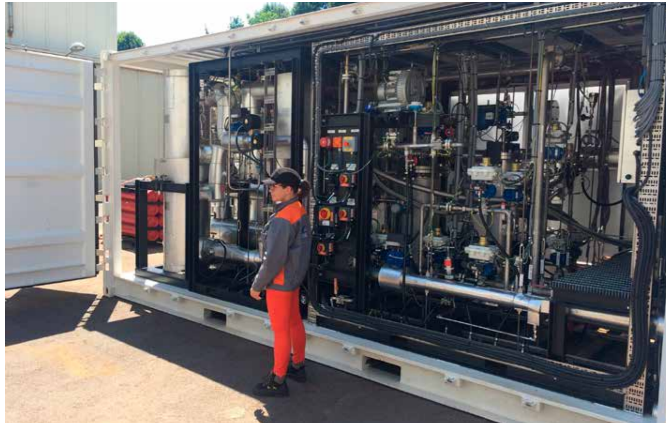
■ The 1MW Pilot GasReformer in Bermeo, Spain.
