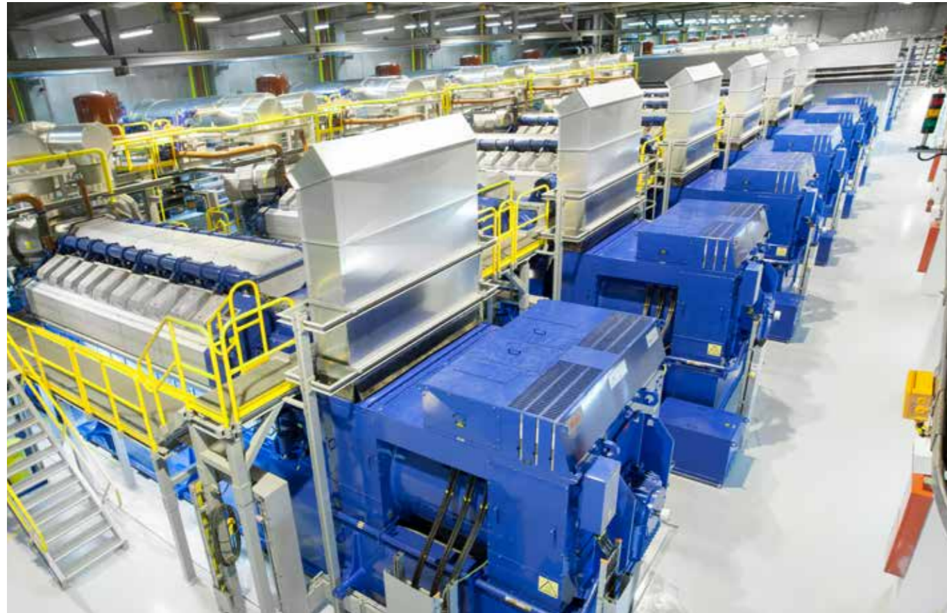
ICE power plants by Wärtsilä comprise several independent 10-20 MW engine units. The modular design ensures high reliability: if one engine is under maintenance, the others are fully operational. Modularity also enables high part-load efficiency, key in balancing renewables.
